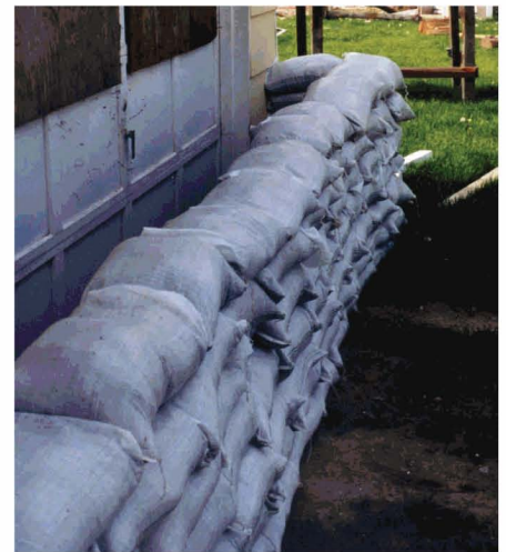
Single stack placement
