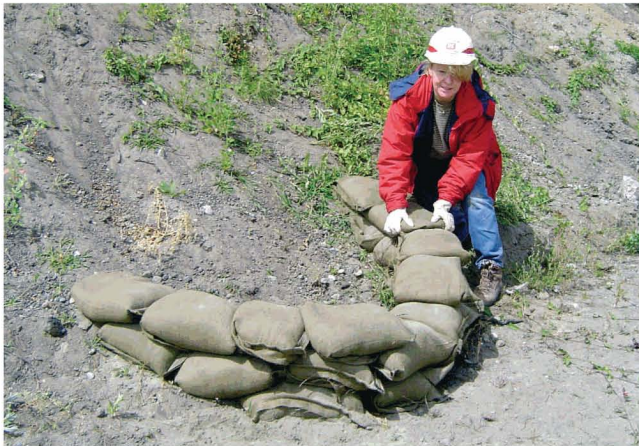
Corps employees demonstrate building a ring dike.
